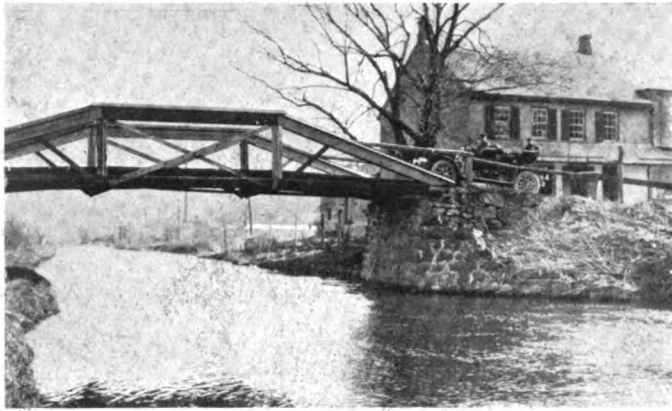
Crossing Old-fashioned Canal Bridge.
